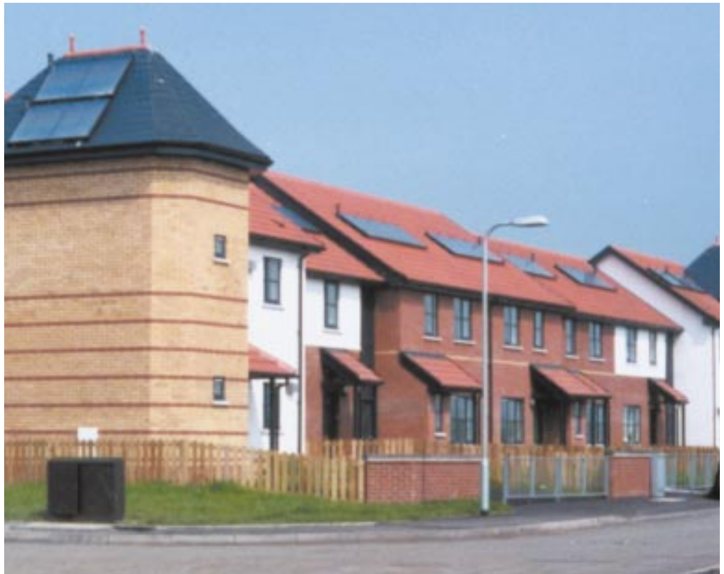
Figure 1 Roof-mounted collectors on Gorseinon development
